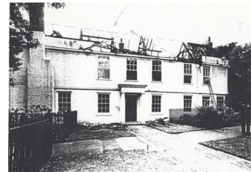
This is a picture of Lauderdale House after the fire in 1963.
